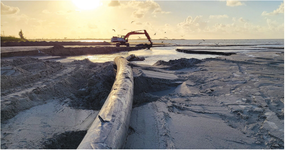
Galveston-Port Bolivar Ferry Dredging. Source: Ecosystem Planning & Restoration
